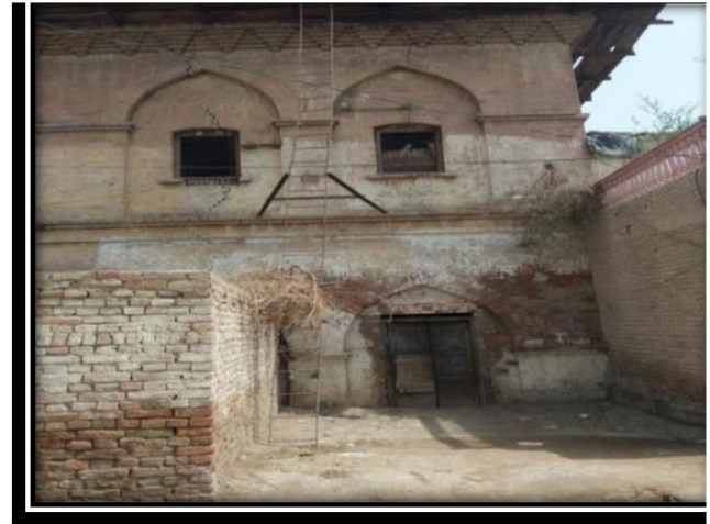
Figure-3: Showing the color of exterior of the Railway colony.
