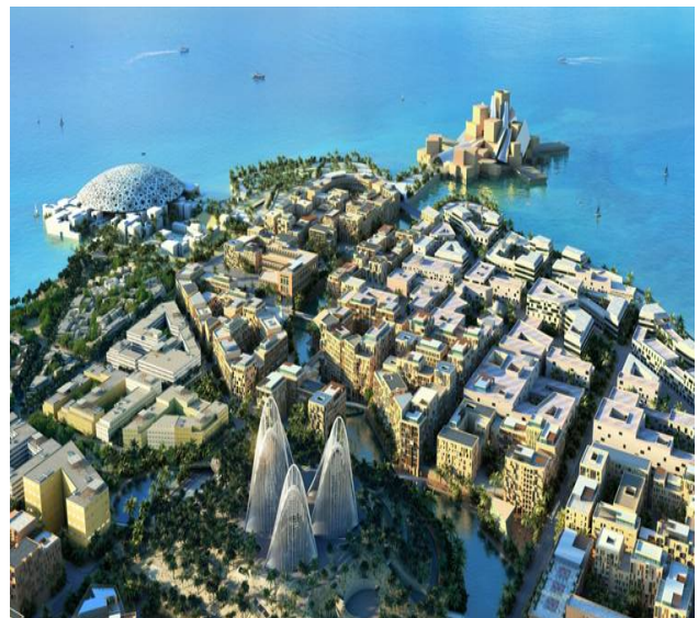
Figure 1: Sadiyat Island Development Project (Saadiyat)
